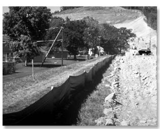
A silt fence is an effective practice for controlling construction site erosion/sedimentation if properly installed and maintained.
